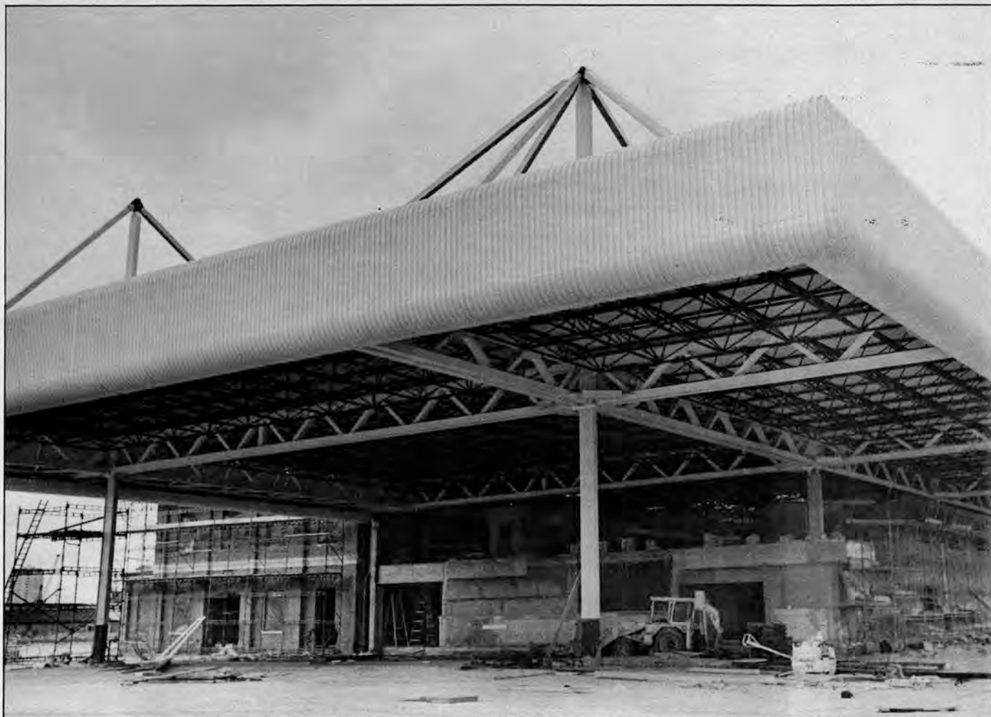
Billingsgate Fish Market in Millwall Docks almost completed. Designed by Newman, Levinson and Partners.
