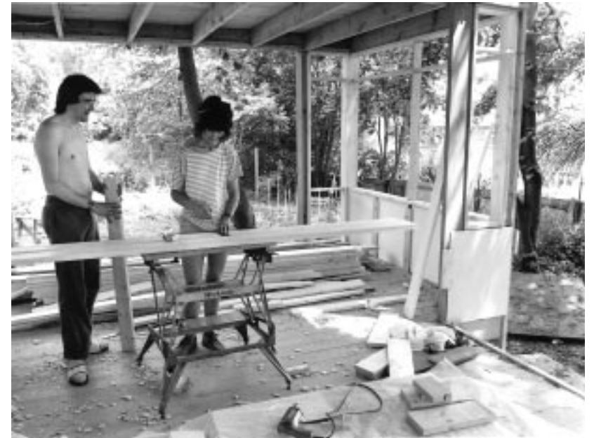
▲ 11 More scope for self-build – timber-frame houses 11–12. Residents on Lewisham Council's housing waiting list build new homes for themselves using a flexible and economical timber-frame design by architect Walter Segal, 1980.
