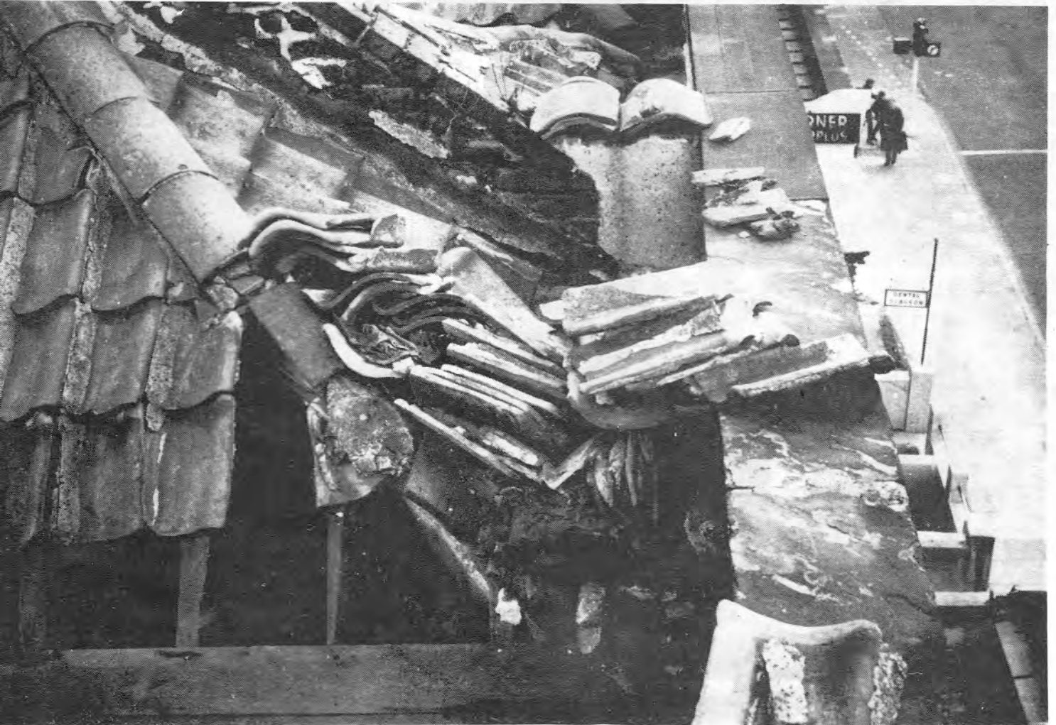
s removed from the roof of a house in Hampstead Road.
