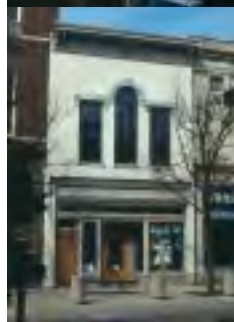
Demonstration project Before and after of a shop used as a neighbourhood planning office and as a demonstration for improving street frontages.
