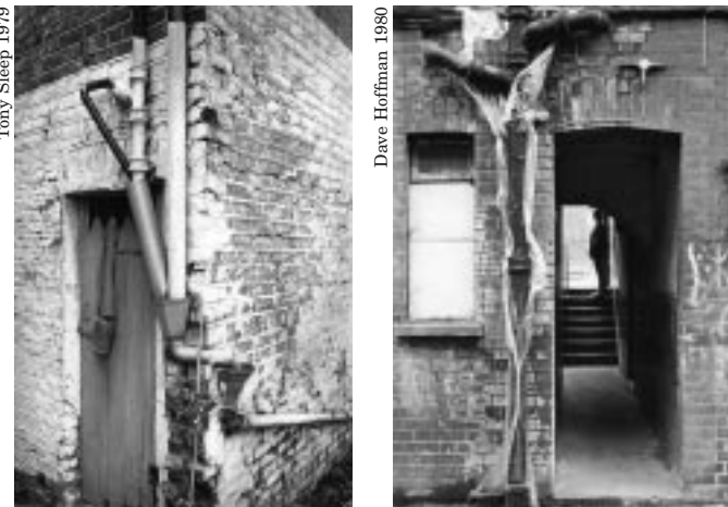
Improvised drainpipes: Freston Road and Fieldgate Mansions
