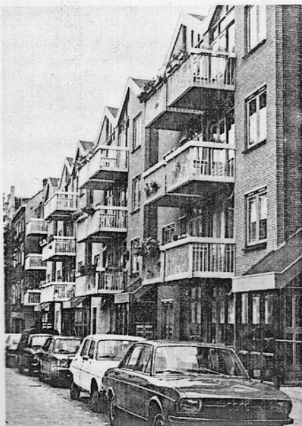
1 Twenty-eight new dwellings in Cool project area, central Rotterdam.
