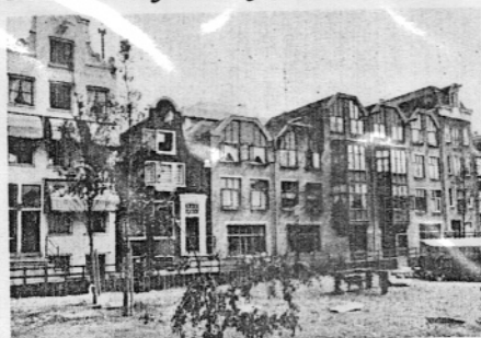
11 Sensitive infill at Bickerseiland. Architect, Paul de Ley.
