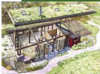
Straw bale construction provides high thermal insulation on an exposed site with a tight budget. Romney Marsh Visitors Centre.
