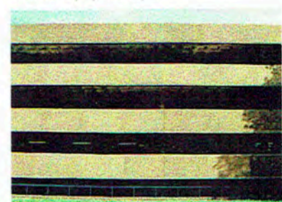
The Westgate car park was often targeted for redevelopment in the long term
